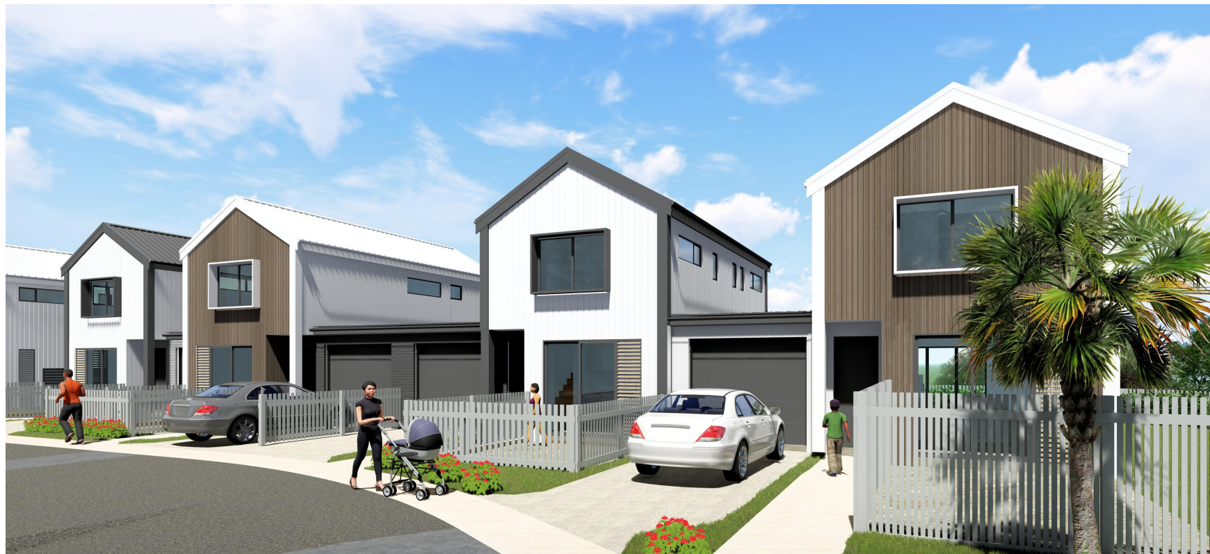
Block A - Rear View
