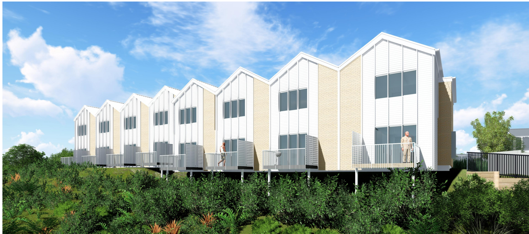
Block E - Rear View
